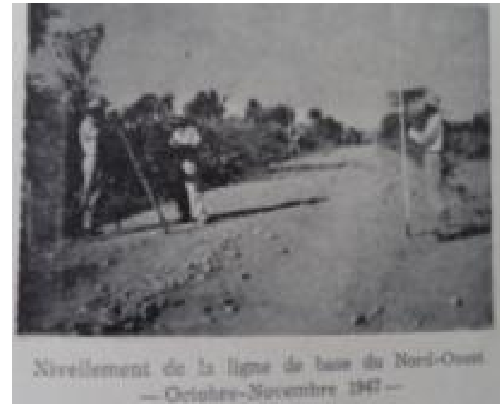
Leveling Measurement, North West , 1947
