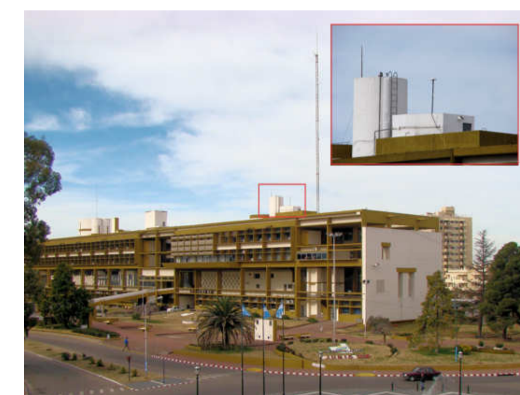
Figure 7: Location of antenna the at Civic Center
